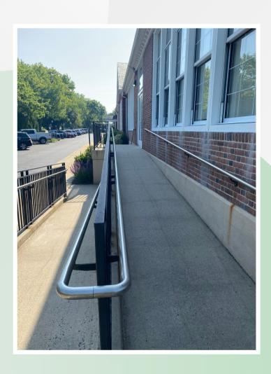
In the spring of 2023, the paving project of the library's circular driveway added wheelchair accessible access to the sidewalk leading to the picnic area and the accessible entrance ramp.
